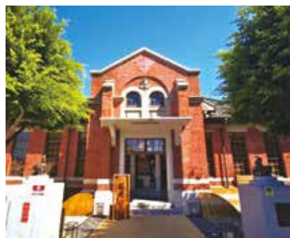
Dounan Police Station Old Office Buildings
